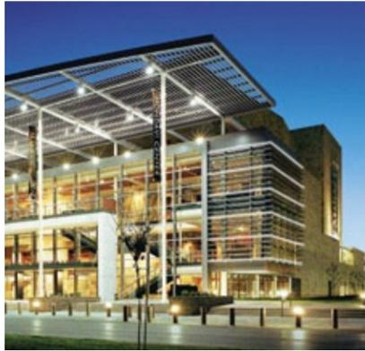
▲ **Concert hall.** Horizontally arranged c|sairfoil® blades have been combined with c|sairfoil LUX® illuminated blades to enhance furthermore the building's impressive illumination at night
